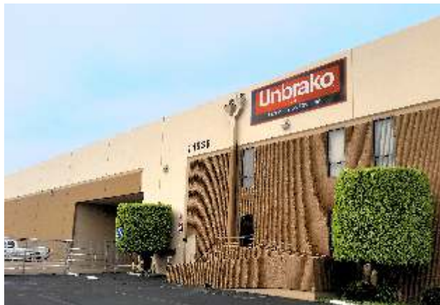
West Coast Distribution Center
